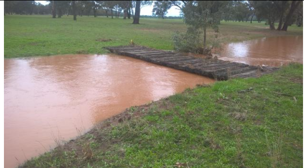
Plate A4.2 – Flooding in the vicinity of the old bridge adjacent to the 4 th fairway of the Bogan Gate Golf Club.
