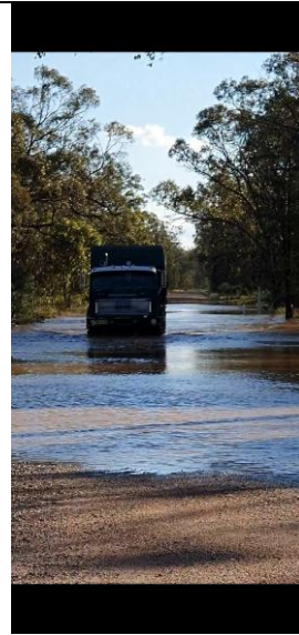
Plate A6.8 – Floodwater inundating the Tubby Lees Road causeway crossing of Gunningbland Creek.
