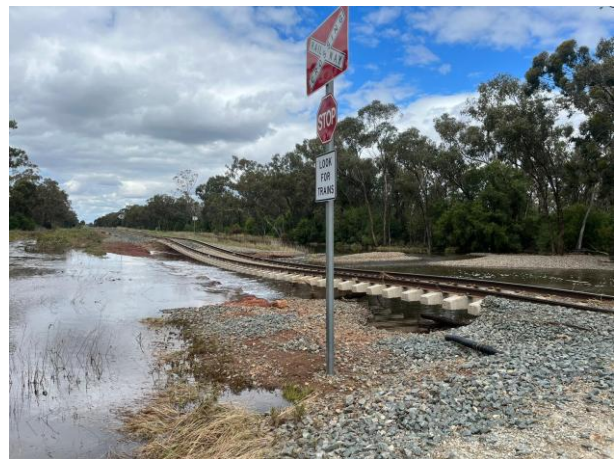
Plate A7.19 – Collapsed section of railway immediately to the east of Overland Road.
