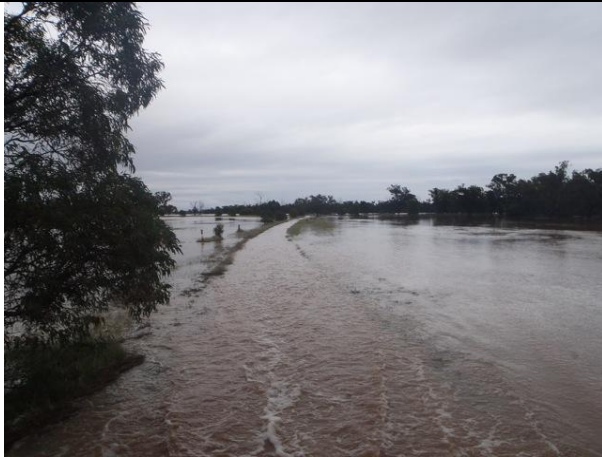
Plate A2.7 – Flooding in the vicinity of the Bogan Gate Golf Club.
