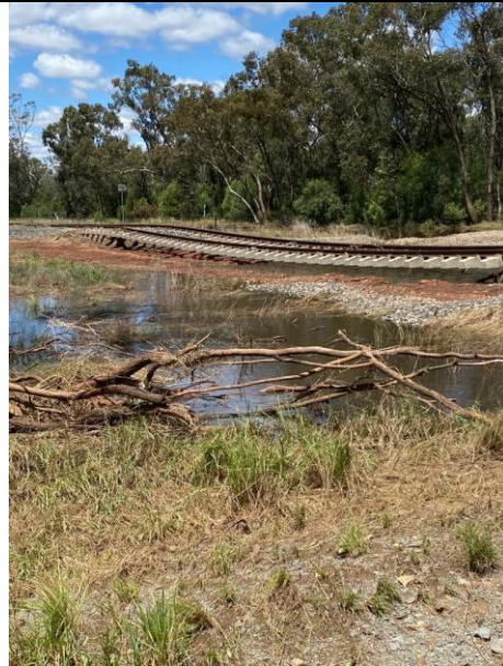
Plate A7.19 – Collapsed section of railway immediately to the east of Overland Road.
