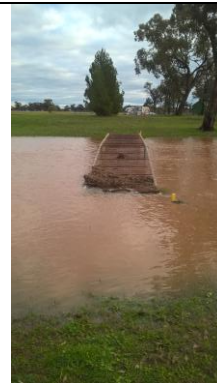
Plate A4.6 – Flooding in the vicinity of the 6 th fairway of the Bogan Gate Golf Club.
